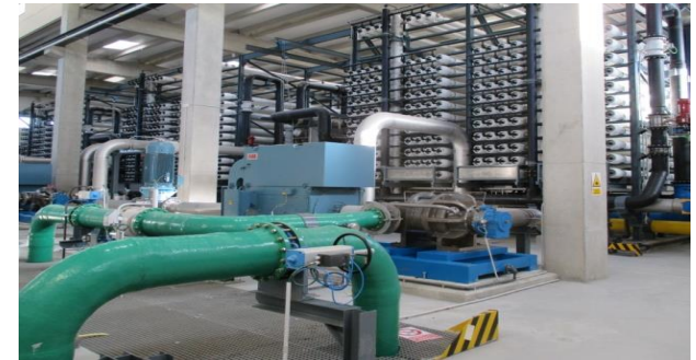
Use of non-conventional resources: desalination plants
