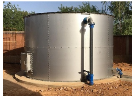
Installation of a raw water tank
