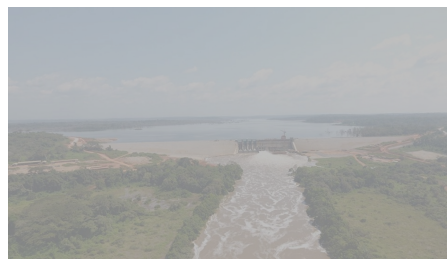
Bassin de la Sanaga © EDC Electricity Development Corporation
