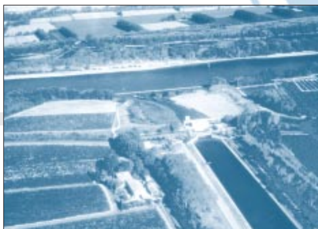
The "Philippe Lamour" irrigation canal in Languedoc (France) - Photo BRL
