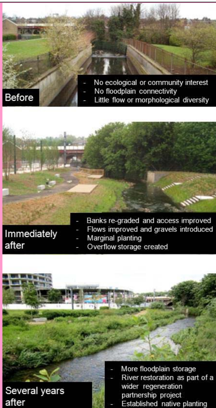
Figure 4.2 River Ravensbourne in south London , before and after its restoration
