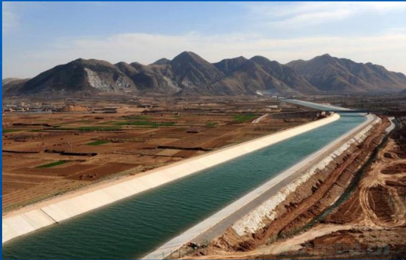
The 3 - 1000 km long water S/N transfers diverting flows of the Yangtze river to provide water to the water stressed cities of Beijing and Tianjin in the Hai river basin.
